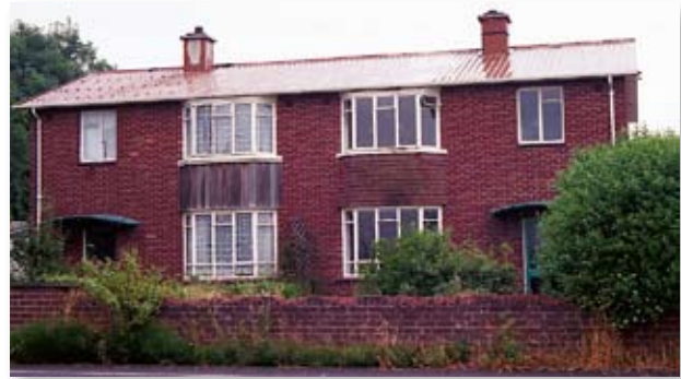
A brick clad experimental aluminium two-storey house at the Brockworth shadow factory site, only one of two built – it is now demolished. Photo: July 1987
